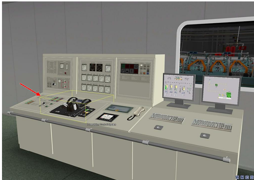
Action screen, example showing the main console in the ECR with selected zoom on the main engine telegraph and propulsion control system
